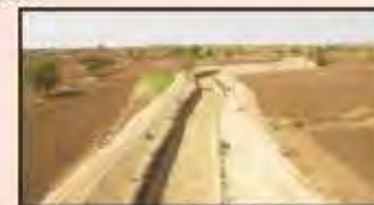
Treatment Work - May 2017
