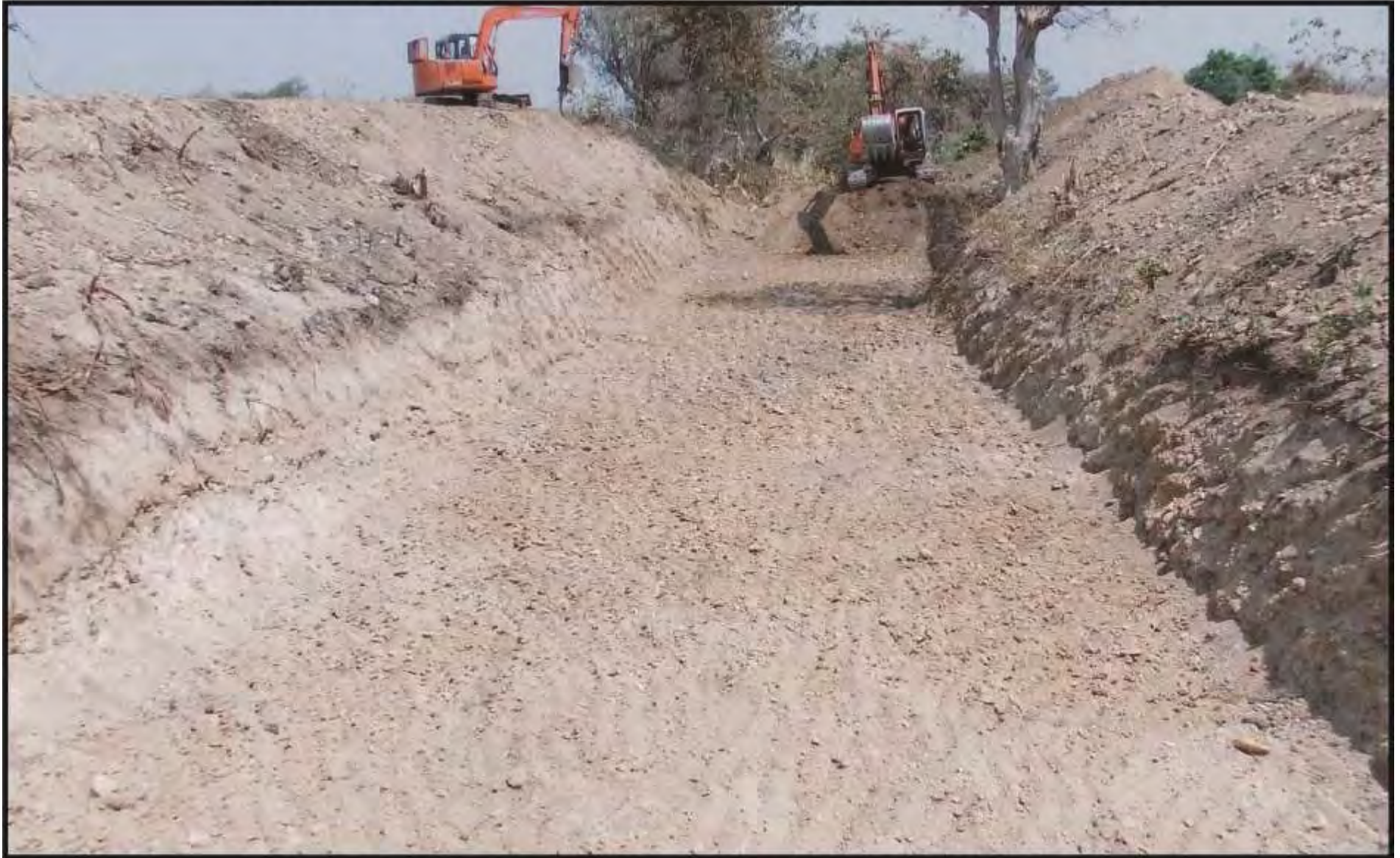
WORK OF DESILTING, WIDENING, DEEPENING OF NALLA BED
