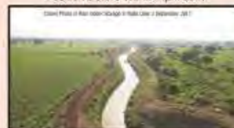
Drone Photo, Storage - 2 September 2017
