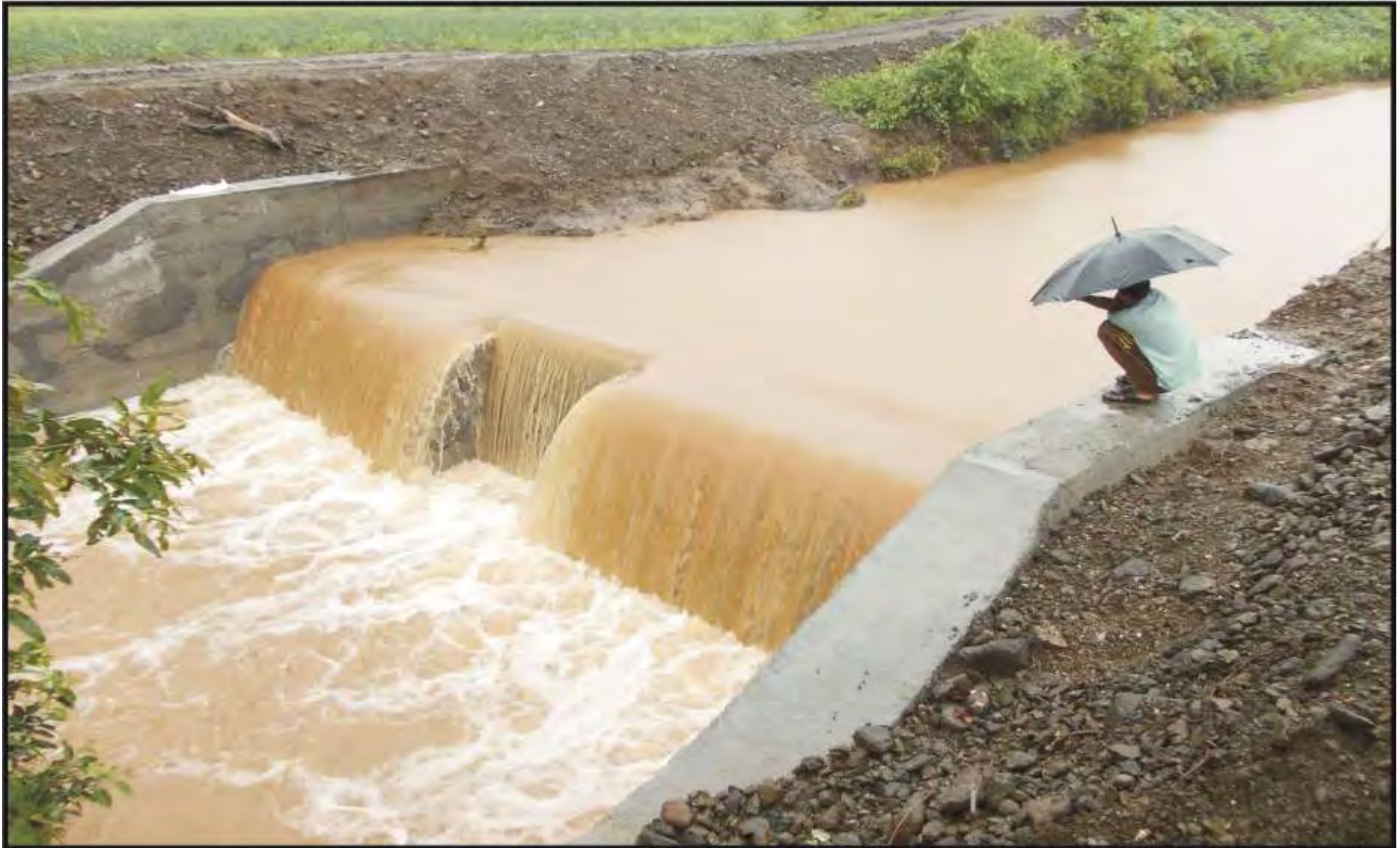
“CEMENT BANDHARA (CHECK DAM) FULL OF RAIN WATER” OVERFLOW FILLING NEXT COMPARTMENT OF NALA
