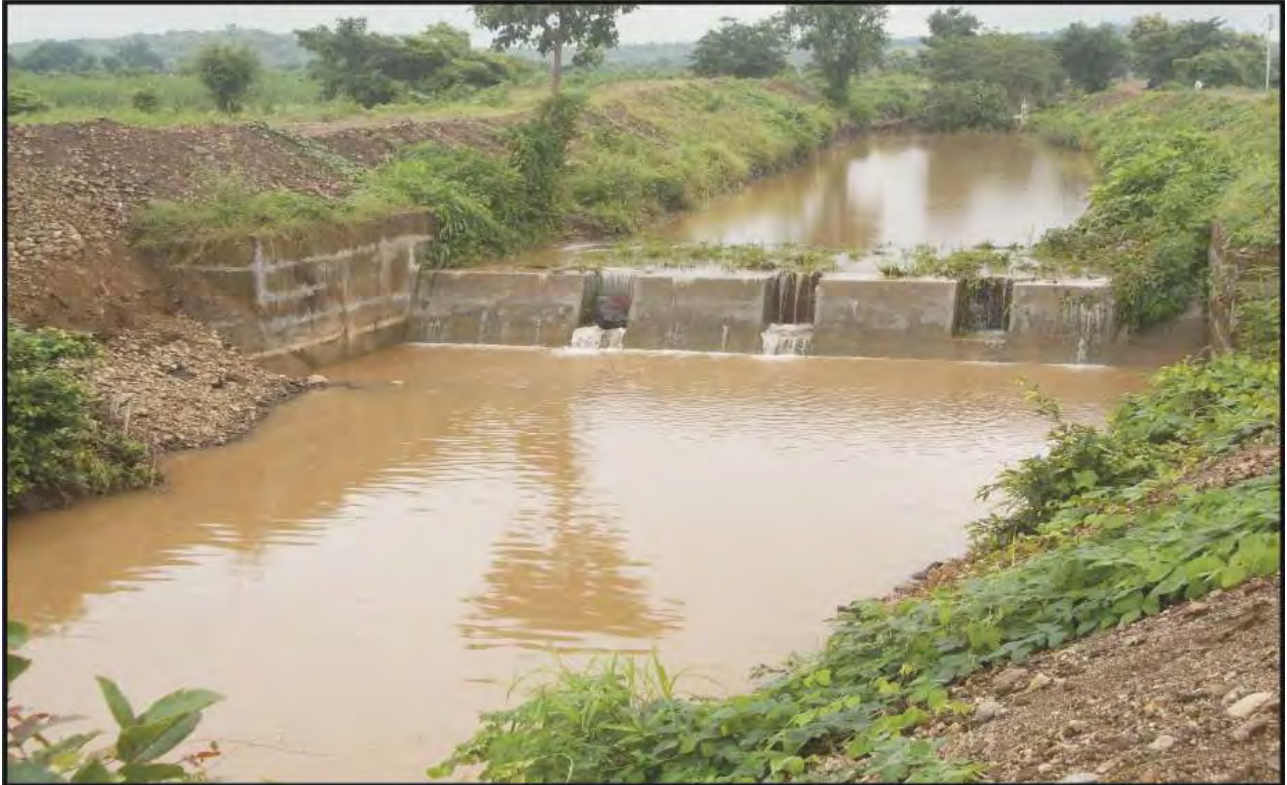
“STORAGE DAM FULL OF RAIN WATER” TOWARDS VALLEY PORTION OF NALA
